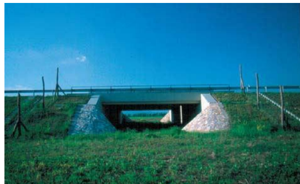
Figure 30 An example of passage below the finished road level in Hungary, designated only for game animals
