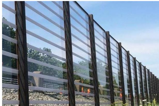
Figure 28 An example of noise barrier with strips that repel birds
